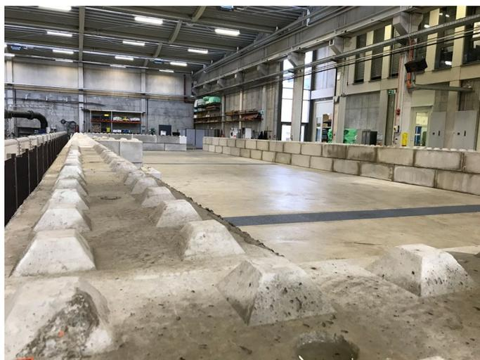
**Fig. 2** Construction work on a physical model of Havel polder. A base frame with a length of 34 m and width of 11 m is set up with concrete building blocks to form a basin; afterwards, a model dike with a breach will be constructed inside. Flooding this structure will give insight into the filling characteristics, so that constructional measures for an intended filling of the polder can be concluded
