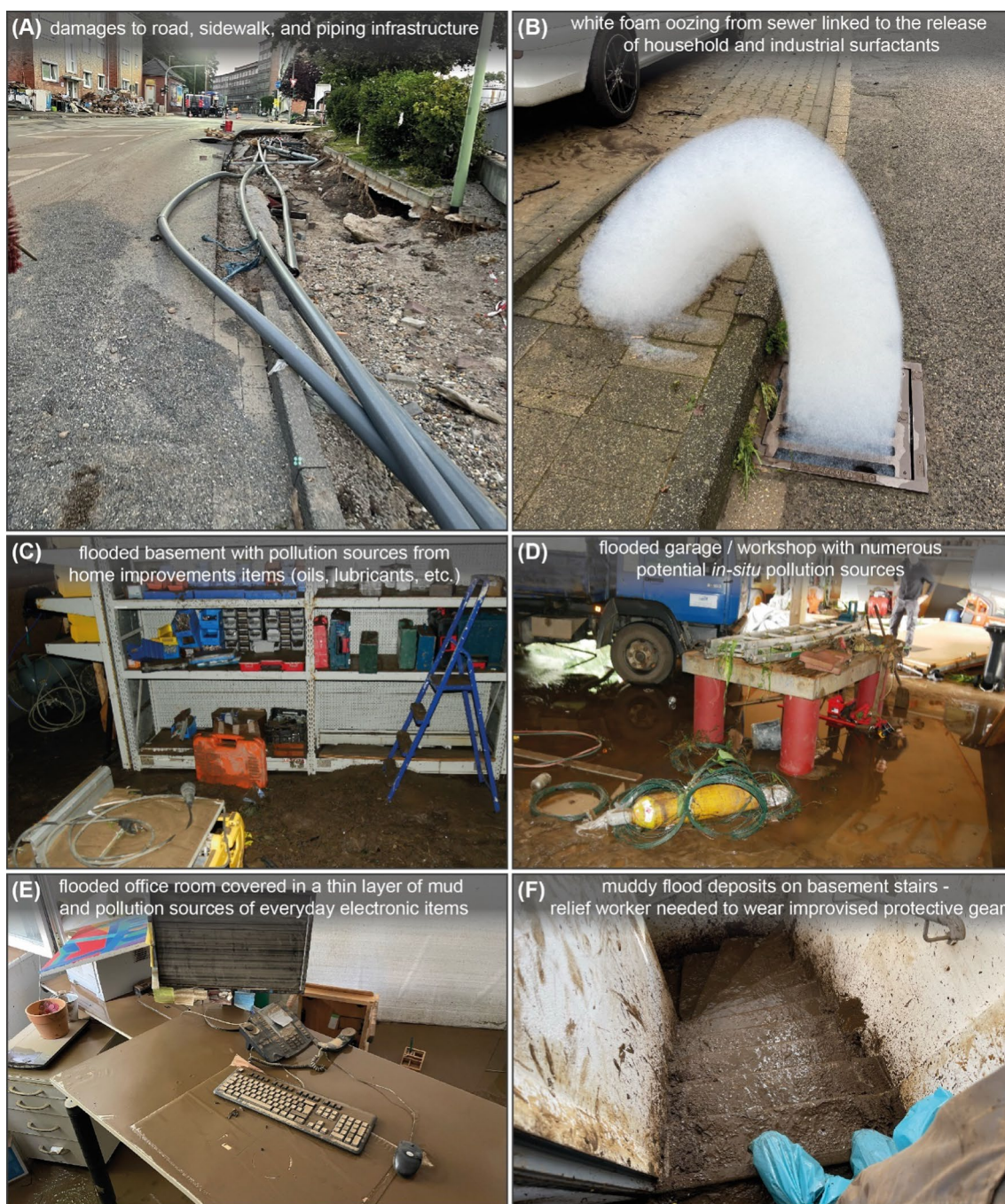
Fig. 7 Photo plate of flood-related damages and pollution sources along the Vicht and Inde rivers. A Damages to a road, erosion of the sidewalk and piping infrastructure in the industrial areas at Zweifaller Straße (L238) in Stolberg. Photo—courtesy of Tristan Lothmann. B Unknown white foam oozing from sewer in the aftermath of the flood. The foam is likely linked to the release of household and industrial surfactants. Photo—courtesy of Tristan Lothmann. C Flooded basement with in situ pollution sources from home improvements items (e.g., oils, lubricants, etc.). Photo—courtesy of Tristan Lothmann. D Flooded garage and workshop with numerous potential in situ pollution sources. Photo—courtesy of Tristan Lothmann. E Flooded office room covered in a thin layer of mud. In situ pollution sources from everyday electronic items and office supplies. Located in a municipal office building at Willy-Brand Platz in Stolberg. Photo—courtesy of Tristan Lothmann. F Muddy flood deposits on basement stairs in Stolberg. First responders and relief workers needed to wear improvised protective gear against hazardous pollution. Photo—courtesy of Tristan Lothmann
