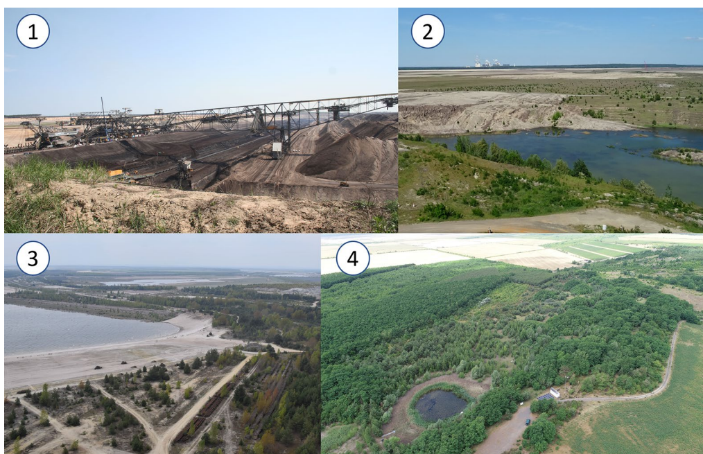
Fig. 3 Operating lignite mining in Lusatia: (1) Active mining operations in the Jänschwalde open cast mine with overburden conveyor bridge F60; (2) emerging new mining lake: The future Cottbus Ostsee as the currently largest artificial lake of Germany is flooded in the former Cottbus-Nord open cast mine. (3) The developing Bergheider See as part of the Lusatian chain of artificial mining lakes. (4) The artificial Hühnerwasser catchment in the Welzow-Süd open cast mine as source for a re-established stream in the post-mining landscape and a scientific research platform for ecosystem research. Photos: F. Lehmkuhl (1, 2013), K. Birkhofer (2, 2018 and 3, 2017), and R. Nenov (4, 2022)
